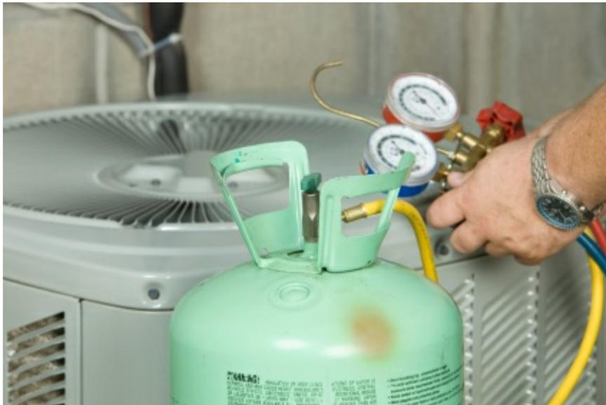
**Incorrect refrigerant levels**— the single most crucial look into preserving your ac unit is ensuring your refrigerant is at the proper level. The refrigerant in your AC is set at installation, and, barring poor setup, having inappropriate refrigerant levels implies you most likely have a leakage.
